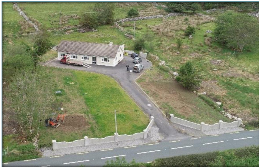
Figure 4b – Drone Shot of the Site (Courtesy of Coyle Environmental)
